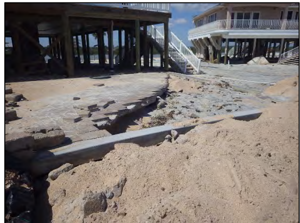
d) Scour under a deck constructed of brick pavers (Latitude 29°40'38.5"N / Longitude 81°12'58.24"W).
