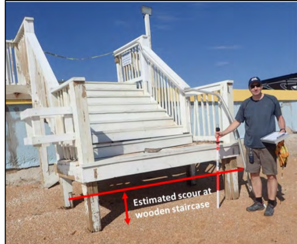
b) Scour at base of timber staircase (Latitude 29°31'14.96"N / Longitude W 81°8'48.07").
