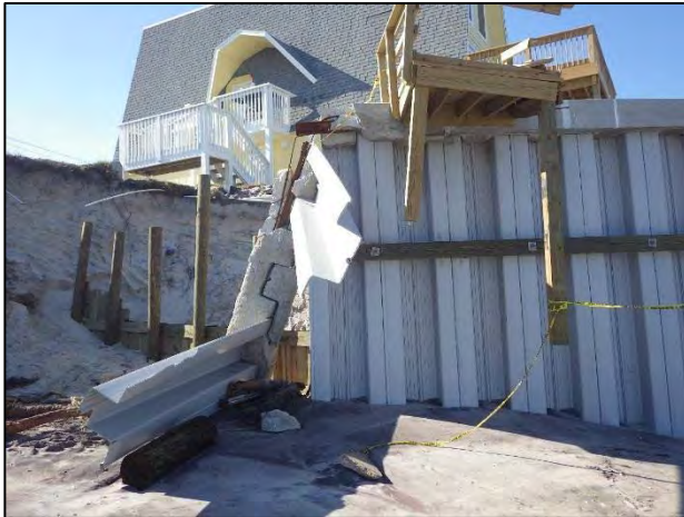
a) South wing wall destroyed.
