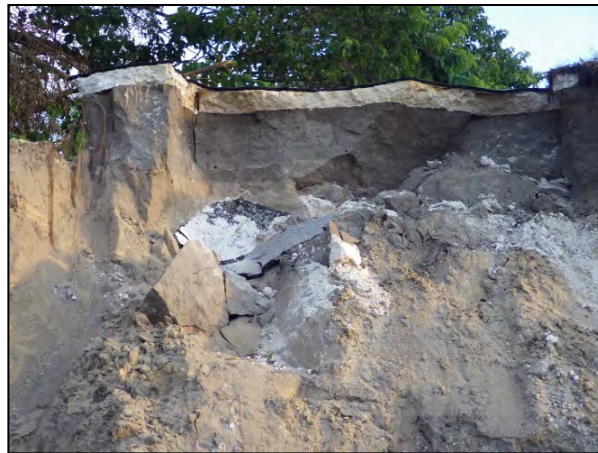
Figure 44. Washout at the West Orange Trail Surface (Latitude 28°41'8.70"N / Longitude 81°30'20.79"W).
