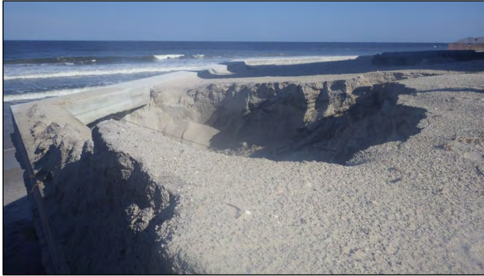
c) Ground loss behind sheet pile (Latitude 29°56'58.16"N / Longitude 81°18'11.96"W).
