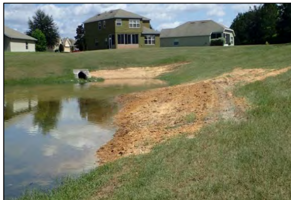
Repaired sinkhole B (back) and C (front)
