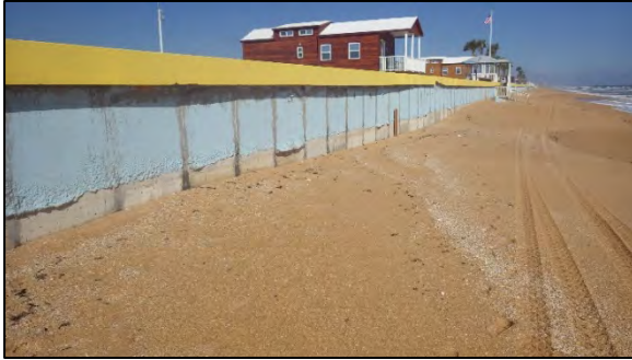
a) Erosion across the face of the wall indicated by the exposed concrete (Latitude 29°31'15.29"N / Longitude 81°8'48.06"W).
