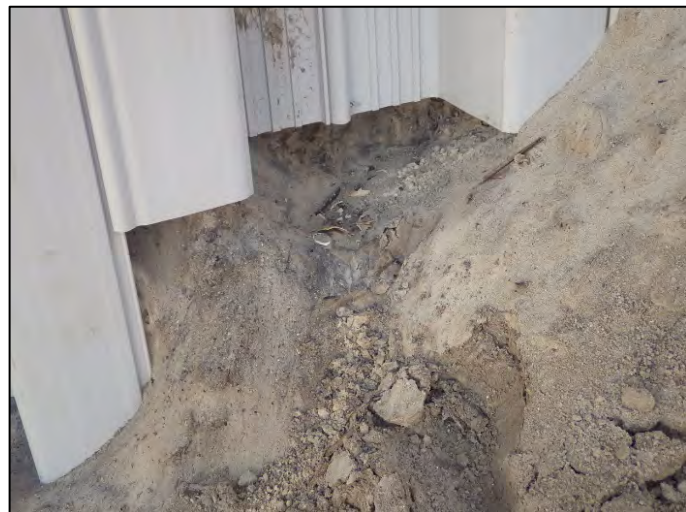
b) Close up of exposed bottom of sheet pile (Latitude 29°56'58.35"N / Longitude 81°18'12.10"W).
