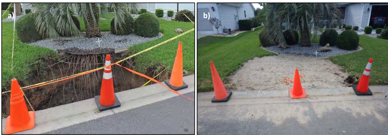
Figure 37. Sinkhole formed at 2532 Botello Avenue a) prior to repair 19 and b) following repair (Latitude 28^{\circ}57'10.60''\text{N} / Longitude 81^{\circ}59'30.50''\text{W} ).
