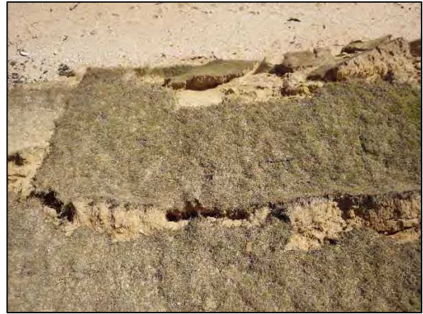
d) Close up of seam in sod where moisture most likely infiltrated into the dune (Latitude 29°32'35.83"N / Longitude 81°9'29.51"W).
