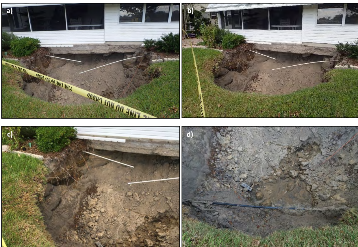
Figure 38. Sinkhole undercutting a foundation at 2536 Botello Rd. showing multiple front views (a, b, c,) and bottom of the sinkhole (d). (Latitude 28^{\circ}57'11.67''\text{N} / Longitude 81^{\circ}59'30.05''\text{W} ).
