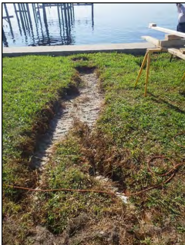
a) Localized scour behind the river bulkhead.
