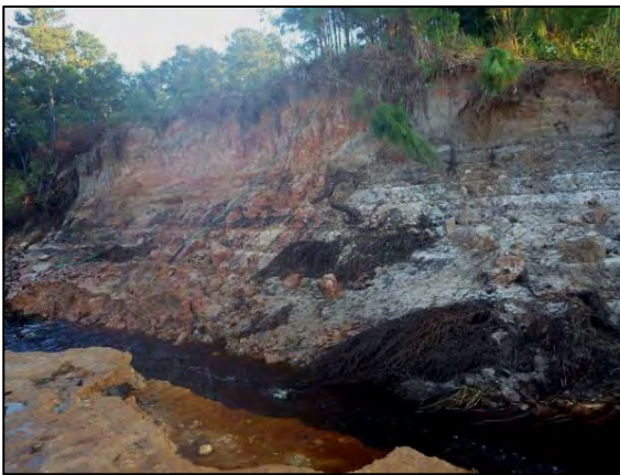
c) Scour of the east embankment of the dam (Latitude 30°46'33.89"N / Longitude 81°58'15.47"W).
