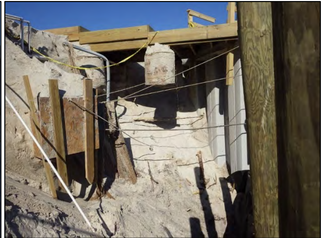
b) Damage behind the retaining structure.
