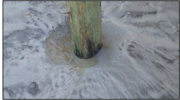
b) Localized scour along pile foundation (Latitude 29°40'57.91"N / Longitude 81°13'5.51"W).
