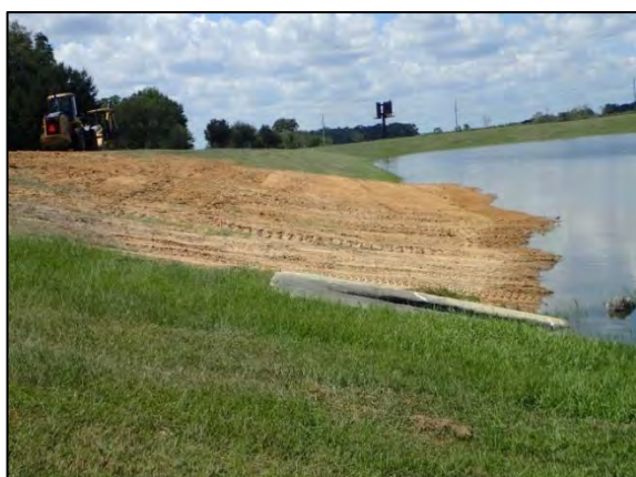
Repaired sinkhole D
