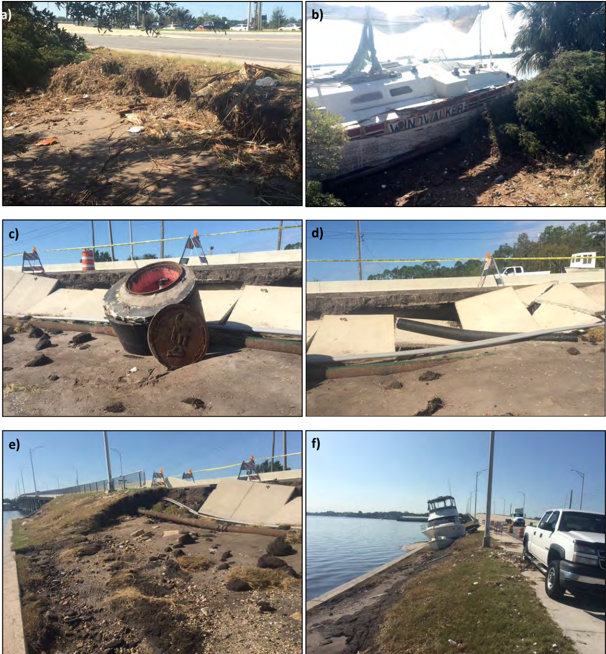
Figure 94. Scour damage along the northeast bridge embankment of the US 17 bridge over the Trout River, (Latitude 30°23'45.44"N / Longitude 81°38'53.95"W). Scour features are presented from north to south toward the concrete cover of the embankment that demonstrate erosion of soil below the road shoulder that resulted in broken pavement and exposed buried infrastructure that included: shallow roadside scour (a); boat washed ashore and scour pattern (b); an exposed sewer access structure and sewer pipe originally located 5 feet below finished grade (c); exposed sewer pipe and conduit for electrical service to light poles (d), and; the terminus of scour (e). Scour was likely caused by eddies and turbulence around two boats washed ashore (f).
