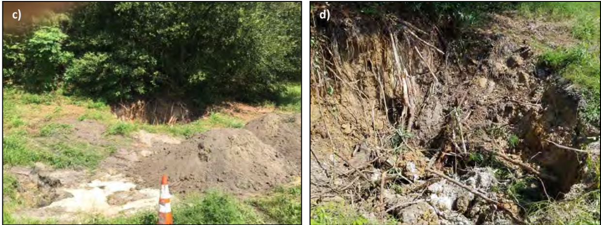
Figure 19: Images of the sinkholes that formed along I-75 northbound south of the SR 26 interchange: a) roadside sinkhole, b) drainage ditch sinkhole, c) sinkhole at the back slope of the drainage ditch, and d) contents of the back slope sinkhole (pers. comm. Binay Prakash, FDOT ).
