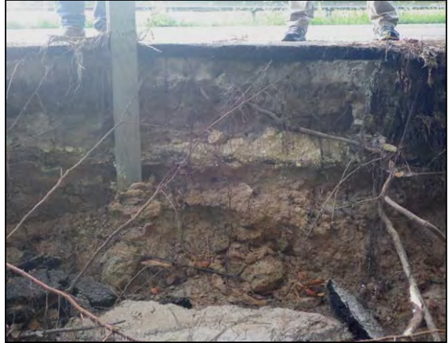
b) Scour at pavement edge on north shoulder of Lake Hampton Road (Latitude 30°46'45.19"N / Longitude 81°58'24.6"W).
