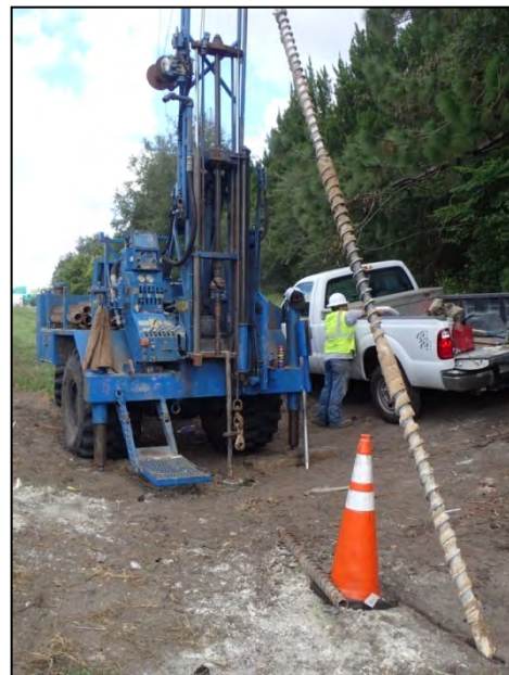
Figure 21: Repair activities for a sinkhole within the drainage ditch off the northbound lane of I-75 with fill and cement grout (Latitude 29°39'8.81"N / Longitude 82°24'45.00"W).
