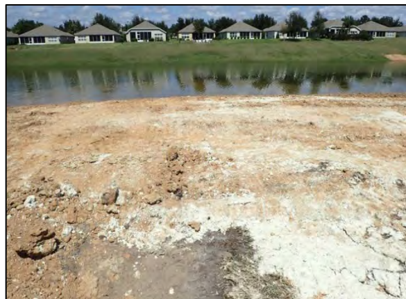
Repaired sinkhole E
