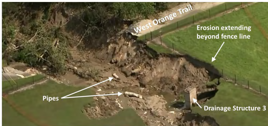
Figure 41: Aerial image of the Apopka erosion washout that bisected the West Orange Trail and damaged two large scale drainage structures 21 (approximate location Latitude 28°41'8.68"N / Longitude 81°30'20.97"W).
