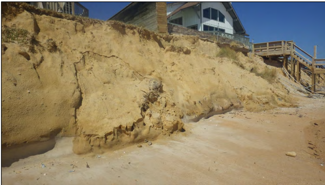
Figure 60. Eroded dune showing active sloughing, undercutting of deck, and potentially unstable timber beach staircase (Latitude 29°32'31.04"N / Longitude 81°9'27.05"W).
