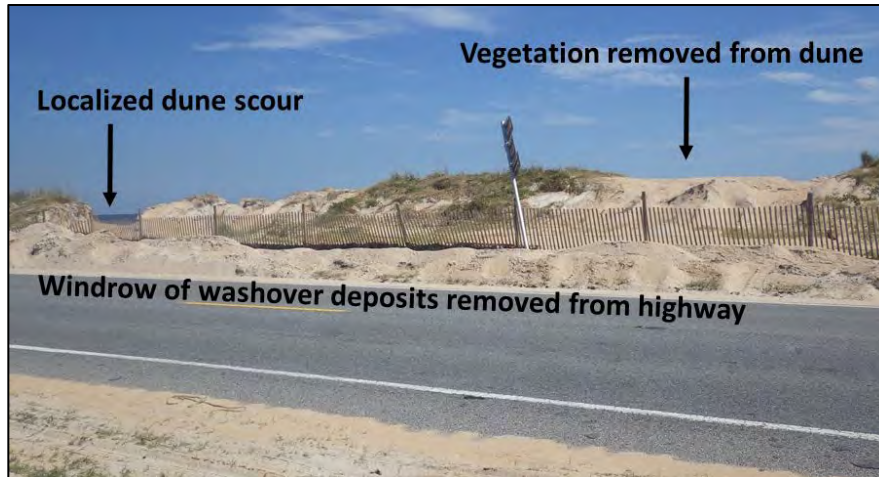
a) Overwash damage to dunes on the east side of Highway A1A (Latitude 29°40'14.09"N / Longitude 81°12'50.37"W).
