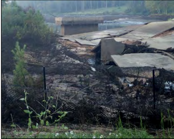
a) Failed dam showing concrete box weir intact (Latitude 30°46'40.1"N / Longitude 81°58'13.0"W).
