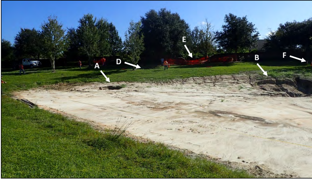
Figure 10: Image of the retention pond showing the locations of wetted clay (left), sinkhole "A", sinkhole "B" with the drainage outfall, sinkhole "D", and sinkhole "E" under the brick wall of the community, and depression "F" (Latitude: 29°40'48.05"N / Longitude: 82°29'43.61"W).
