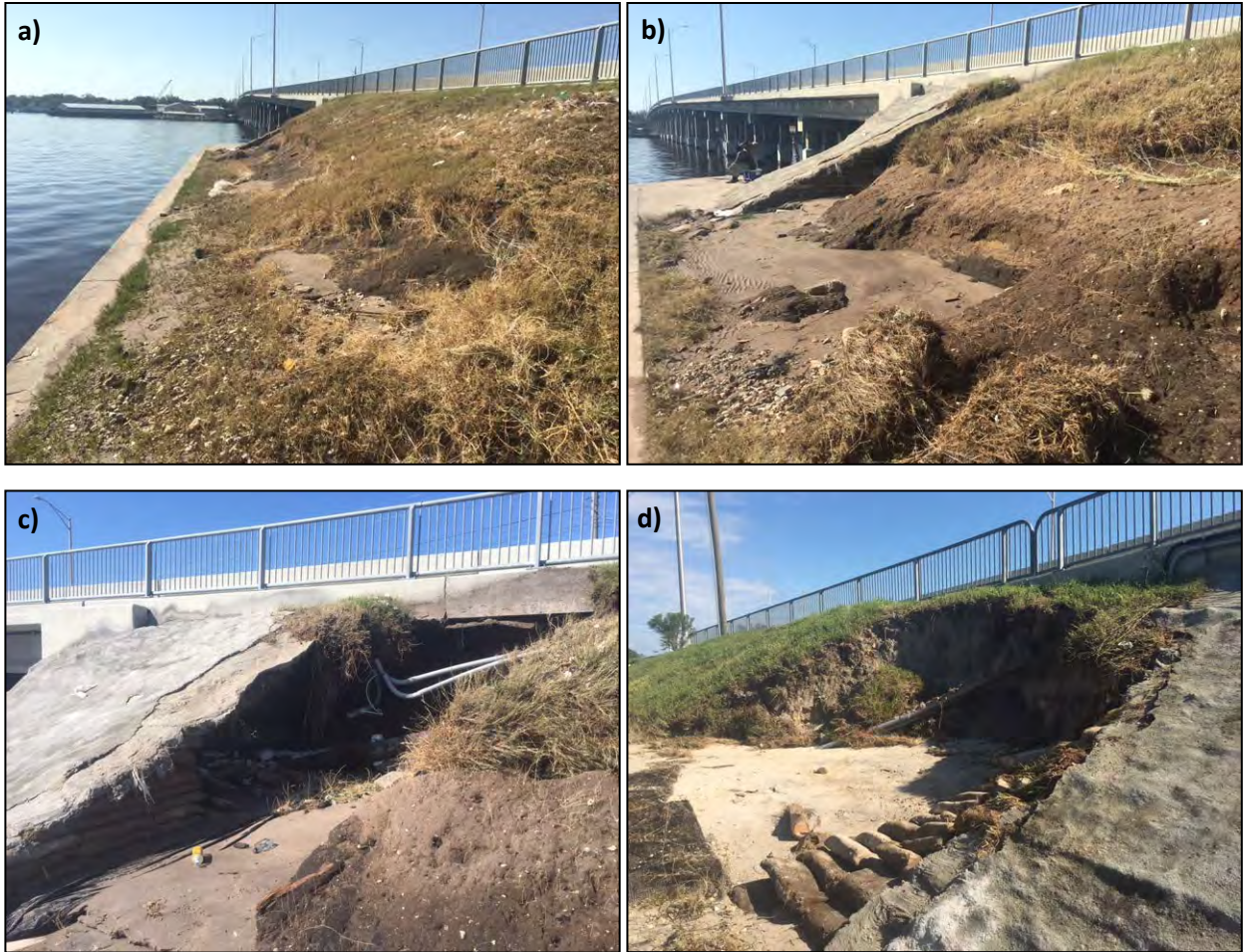
Figure 95. Scour damage along the northern bridge embankment of the US 17 bridge over the Trout River, (Latitude 30°23'44.43"N / Longitude 81°38'54.13"W). Scour features are presented from north east to north west near the concrete cover of the embankment that demonstrate erosion, which included: embankment soil erosion north of the bridge abutment (a, b), and erosion at the interface between the soil and concrete faced, stacked concrete sack wall at the east (c), and west (d) side of the north abutment.
