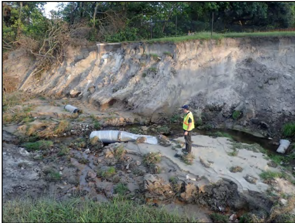
Figure 49. Damaged pipes, eroded West Orange Trail, and uprooted trees at drainage structure 3 area (Latitude 28°41'9.15"N / Longitude 81°30'21.64"W).
