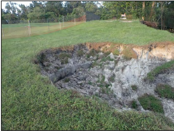
Figure 47. Erosion lateral to the main channel likely from failed drainage structure 3 (Latitude 28°41'9.15"N / Longitude 81°30'21.64"W).
